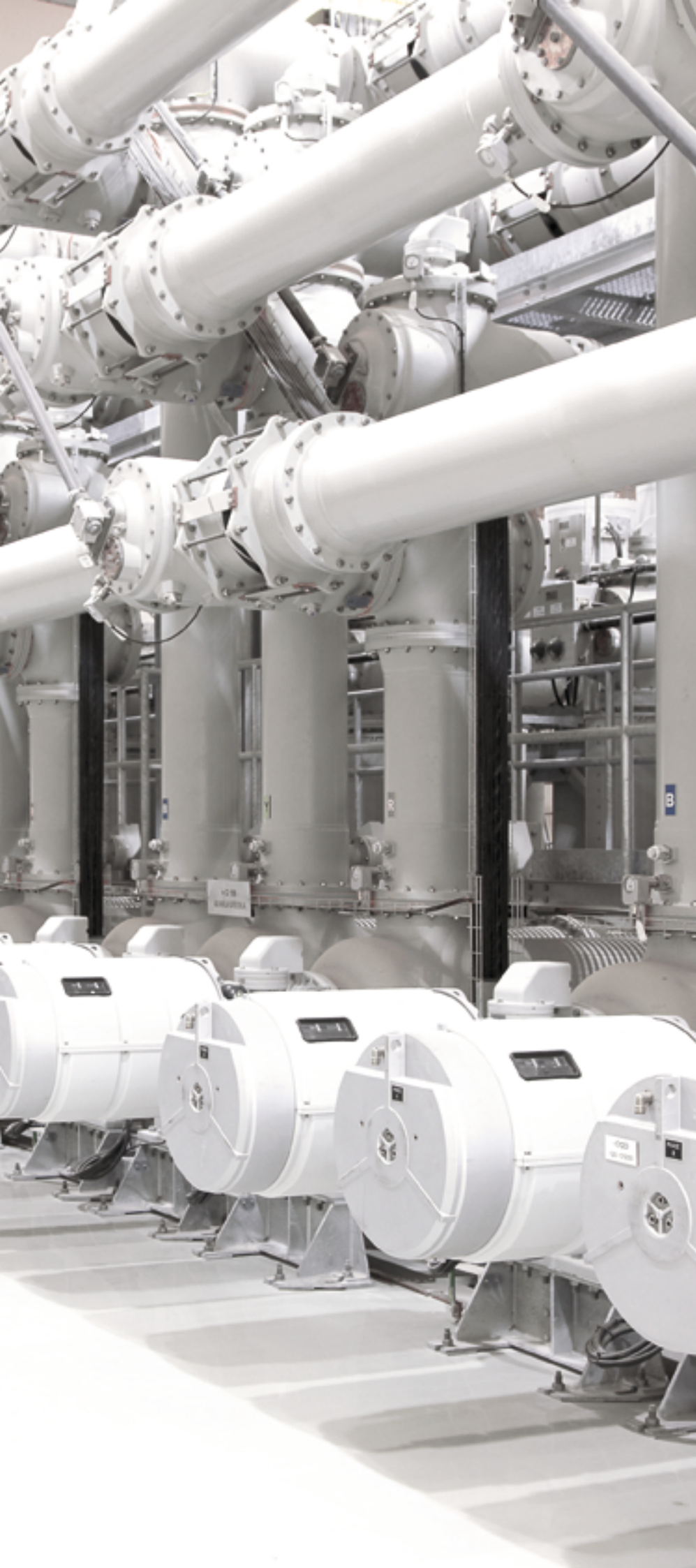
Gas-insulated switchgear (GIS) 400 kV, Qatar 2009 © Hitachi Energy
